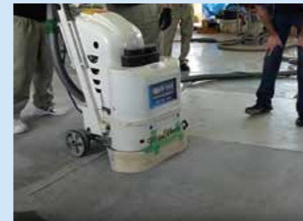
研削~粗研磨 #15~#100 (2~3工程)
